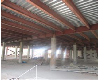
External photo(s) of the production unit(s) 1st floor under construction.JPG
