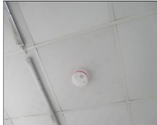
External photo(s) of the production unit(s) Smoke detector.JPG
